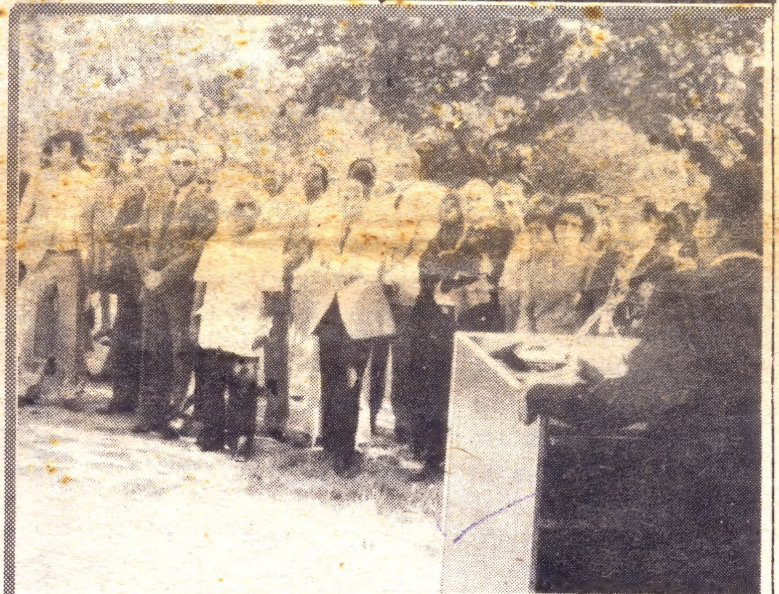
PALM BEACH The OFFICIAL RENOVATION of the ARUBA CARIBBEAN HOTEL took place last Tuesday April 16. During this Renovation 250 Persons will be employed. And then when is finish 400 persons will be employed in the Hotel.
